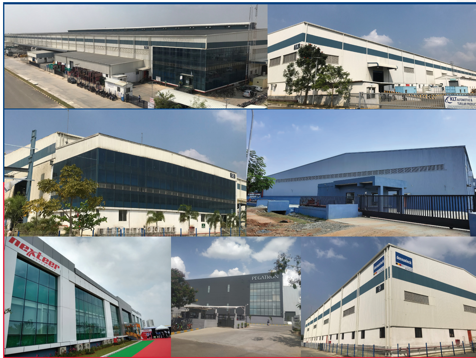
Do My Home | 14,500-sqft 2016 Delivered Manufacture Facility
