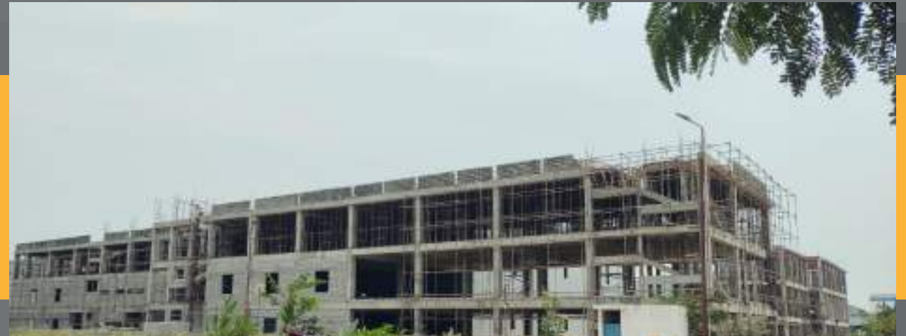
RCC Block : Construction Progress ( Ready by 01/08/2023)
