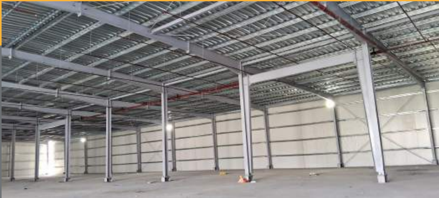
Hall-3 FF fire sprinkler header line and Branch line installation work completed and position welding under progress.
