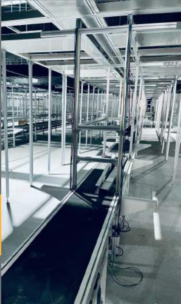
ESD FLOORING READY
