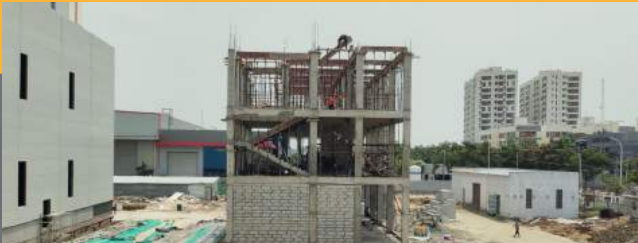
Yard Development + office Block : construction Underway : target Completion : 15/08/2023
