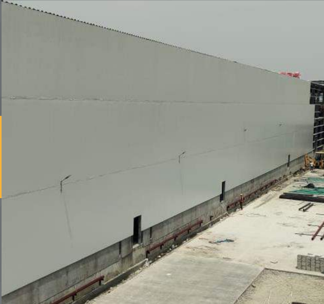
Production Block : Construction Progress ( Ready by 01/07/2023)
